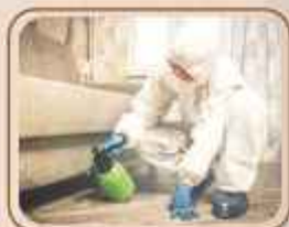
Anti Termite Treatment
