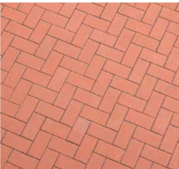
Terrace Brick Bat Coba or Water Proofing Treatment
