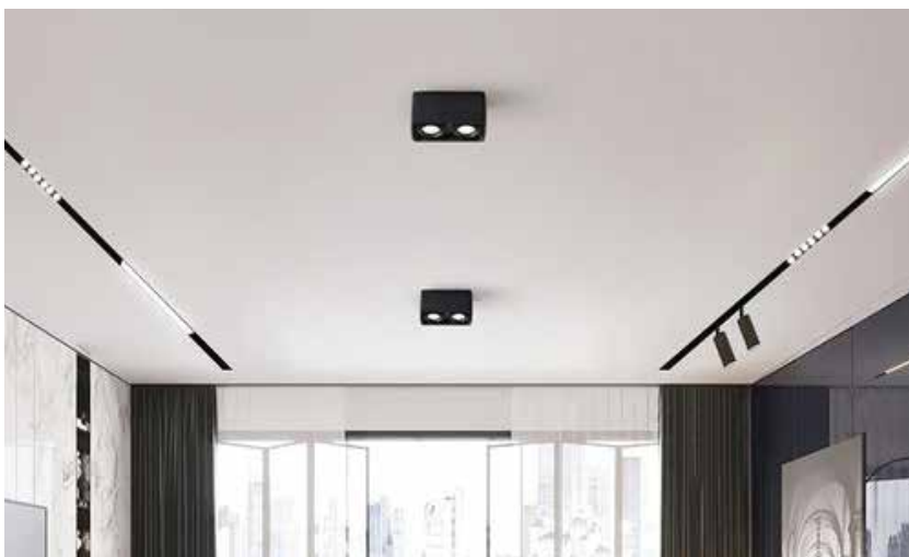
Ceiling Oil Bond Distemper
