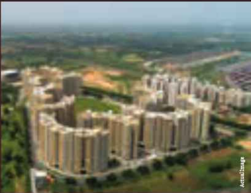
SHANTIGRAM Ahmedabad, Gujarat
